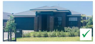
ARTICULATION - the façade addressing the street is to provide visual relief by breaking down the façade into smaller sections. No single wall is to exceed 9 metres in length.
