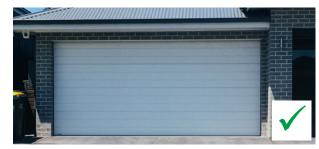
GARAGING – the garage door is not to be a dominant feature of the façade. The garage is to be a maximum of 50% of the width of the façade and is to be set-back a minimum of 1 meter from the main wall of the façade.
